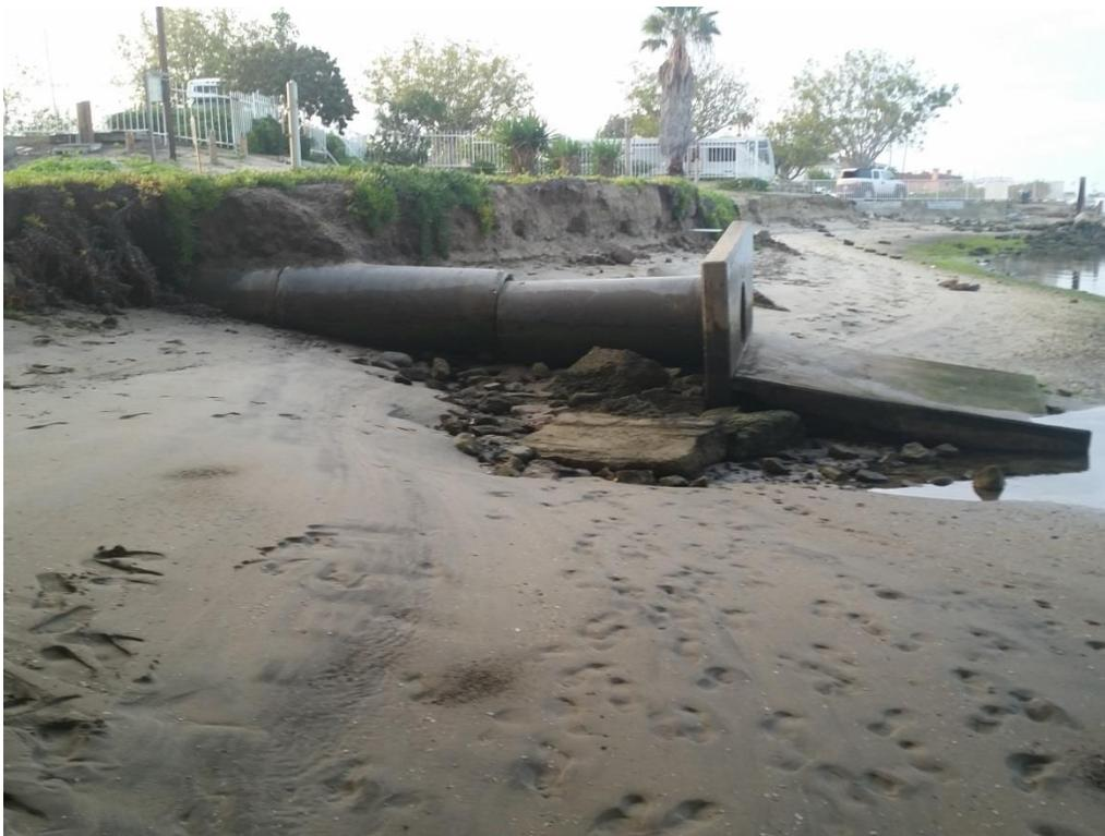
Figure 2 - Existing pipe in forced main crossing south of Bay Bridge, on west side of channel. View to the south.
