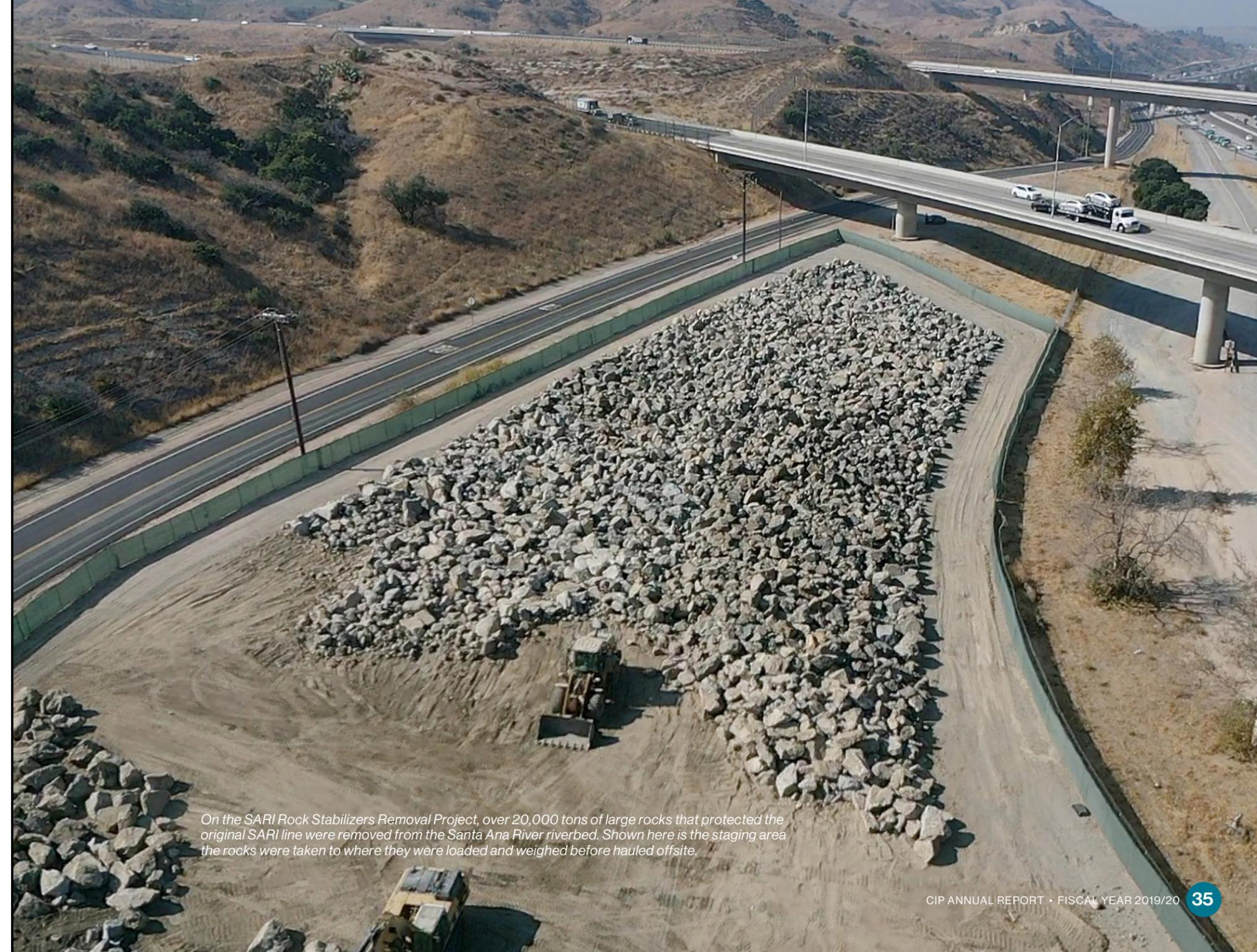
On the SARI Rock Stabilizers Removal Project, over 20,000 tons of large rocks that protected the original SARI line were removed from the Santa Ana River riverbed. Shown here is the staging area the rocks were taken to where they were loaded and weighed before hauled offsite.
