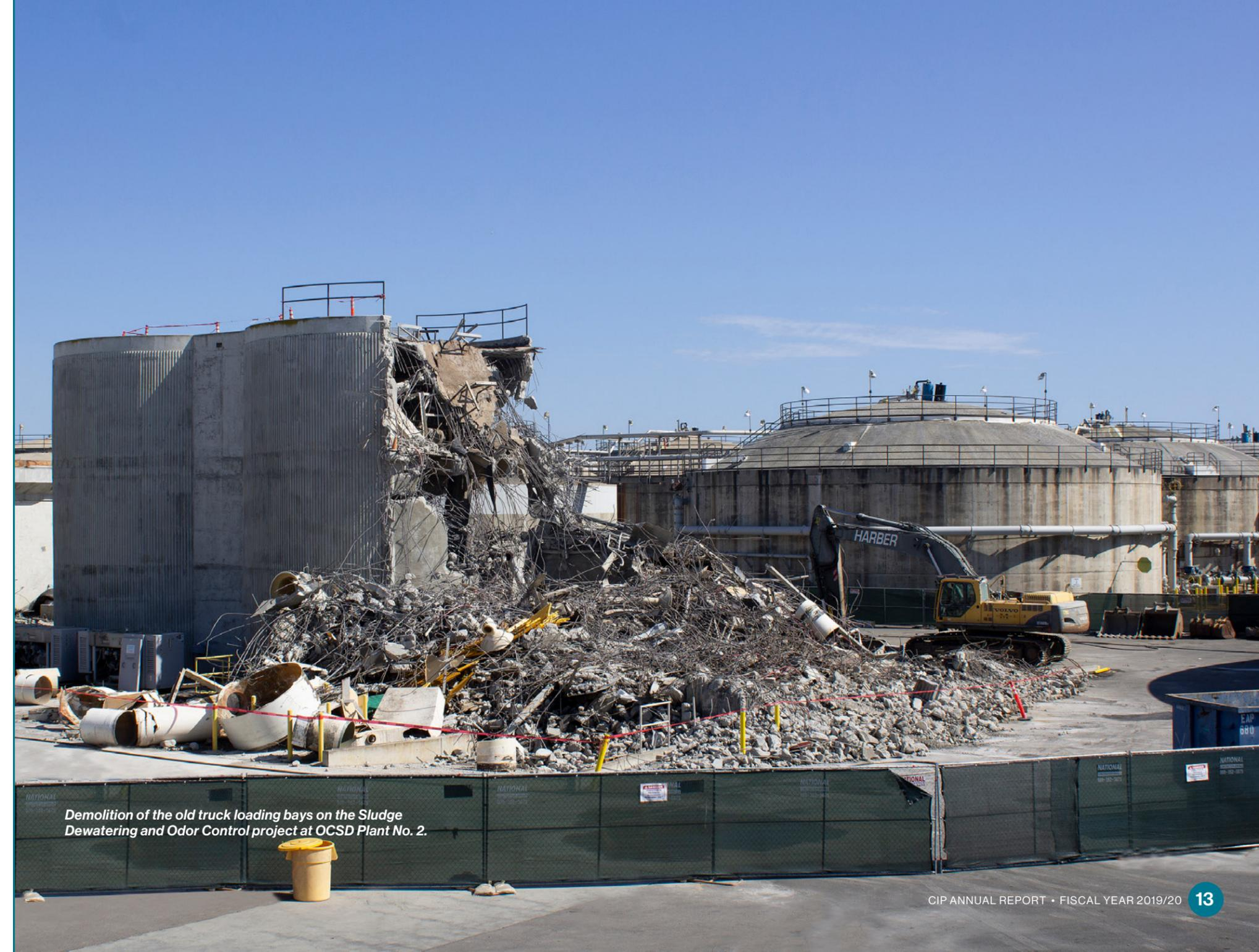
Demolition of the old truck loading bays on the Sludge Dewatering and Odor Control project at OCSD Plant No. 2.
