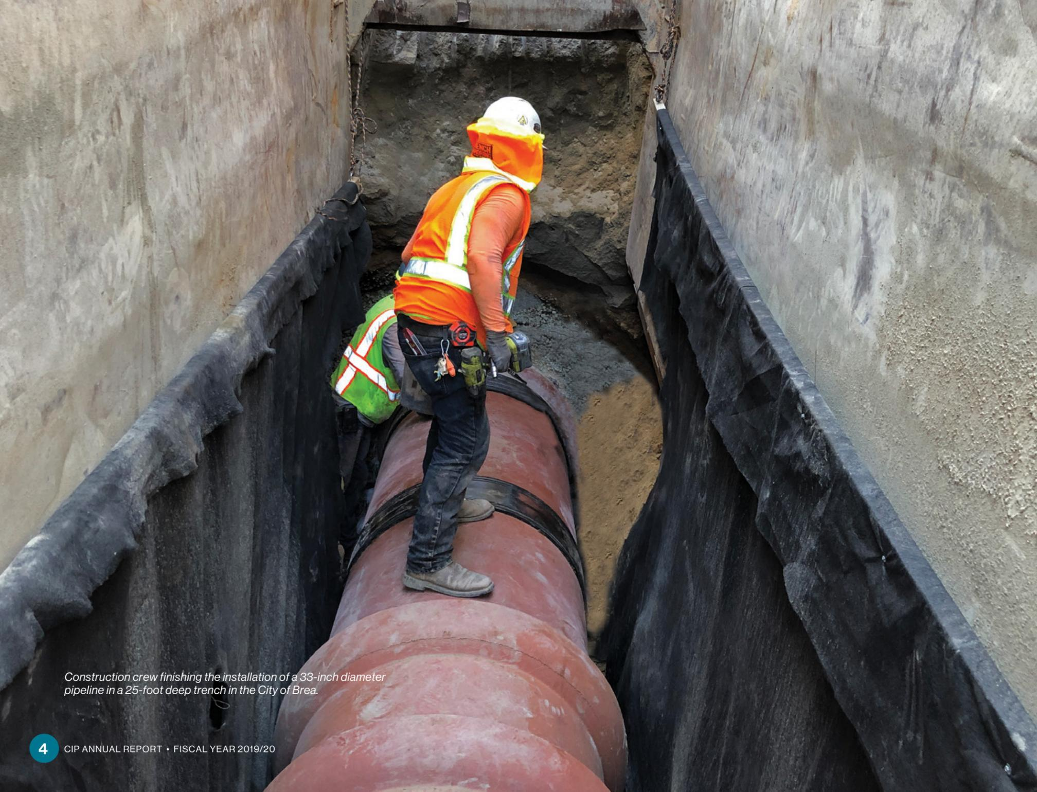
Construction crew finishing the installation of a 33-inch diameter pipeline in a 25-foot deep trench in the City of Brea.
