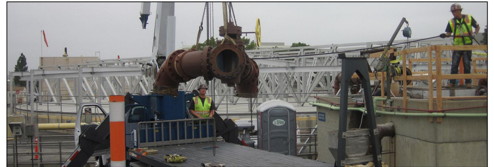
Plug valve being set on a flatbed truck on the East Basin Distribution Box Repair at OCSD Plant No. 1.
