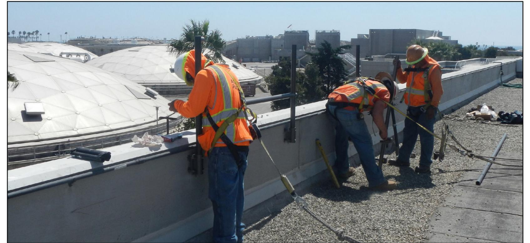
Guardrails are being installed at the OCSD Plant No. 2 Maintenance Building as part of the Safety Improvements Program.
