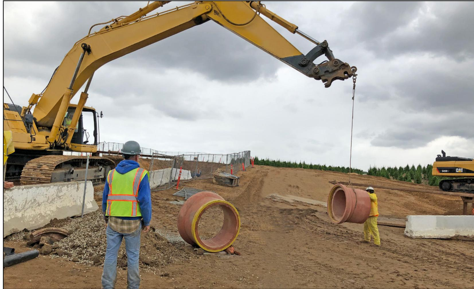
A backhoe lifts a 2-foot long piece of pipe on the Carbon Canyon Pipeline Sag Repairs project in the City of Brea.
