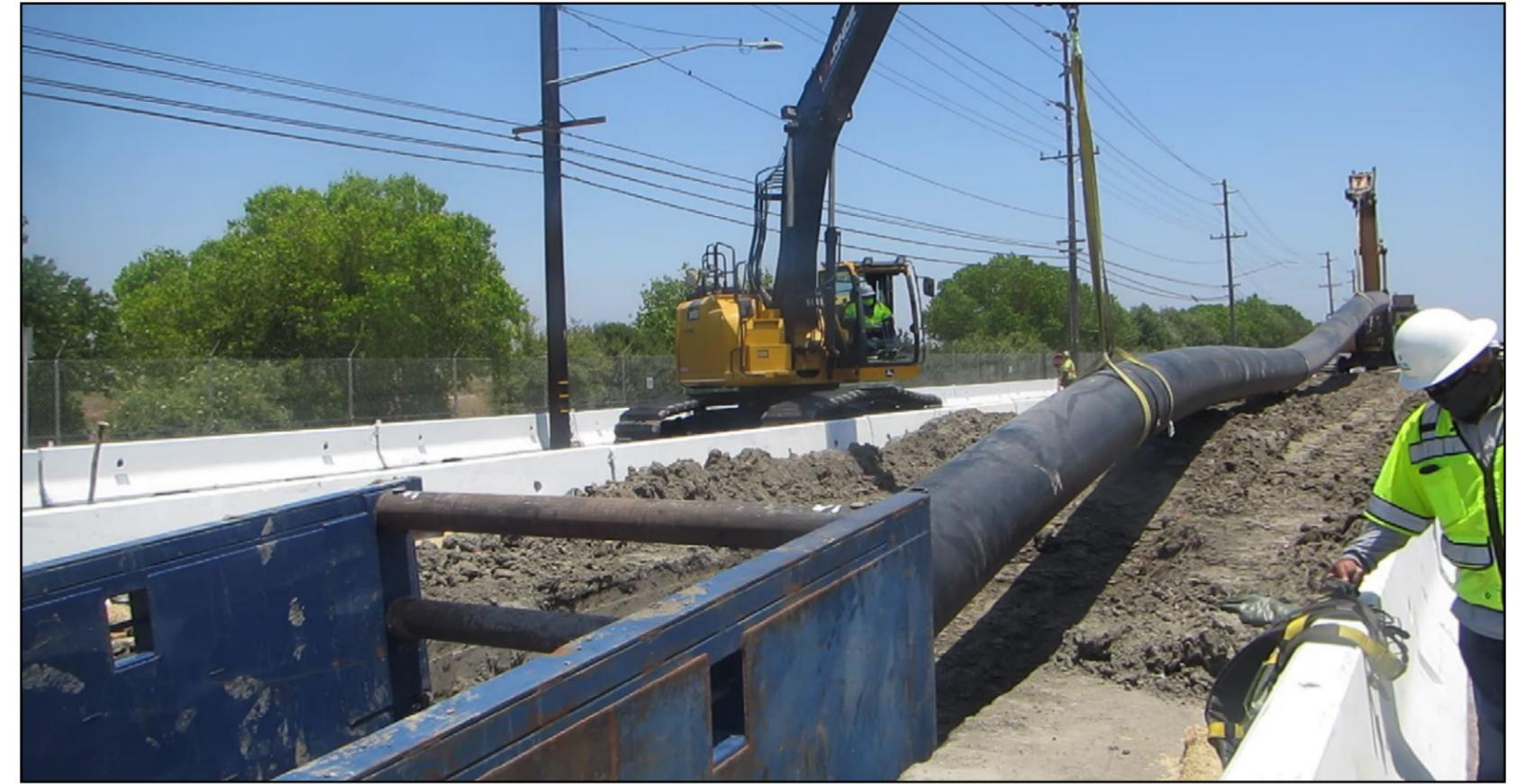
Two excavators are used to install a 200-ft section of a new 36-inch diameter force main within the 10-ft deep trench excavation on Westminster Boulevard in the City of Seal Beach.
