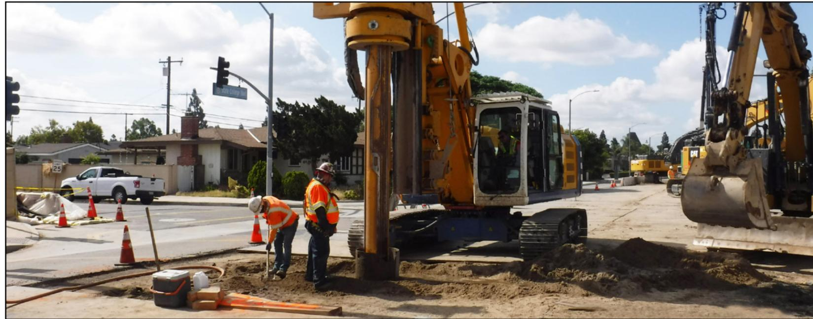
Construction crew is shown pre-drilling a shoring beam on State College Boulevard in the City of Anaheim.
