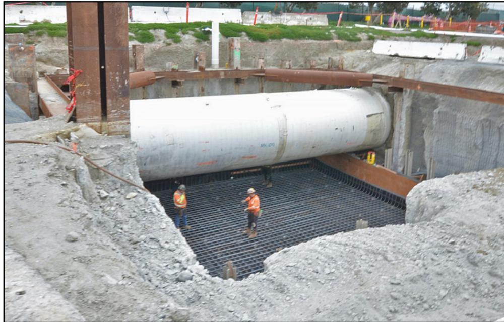
*Excavation and shoring over the 120-inch diameter secondary effluent pipeline at OCSD Plant No. 2 in preparation for the plant water pump station junction structure.*
