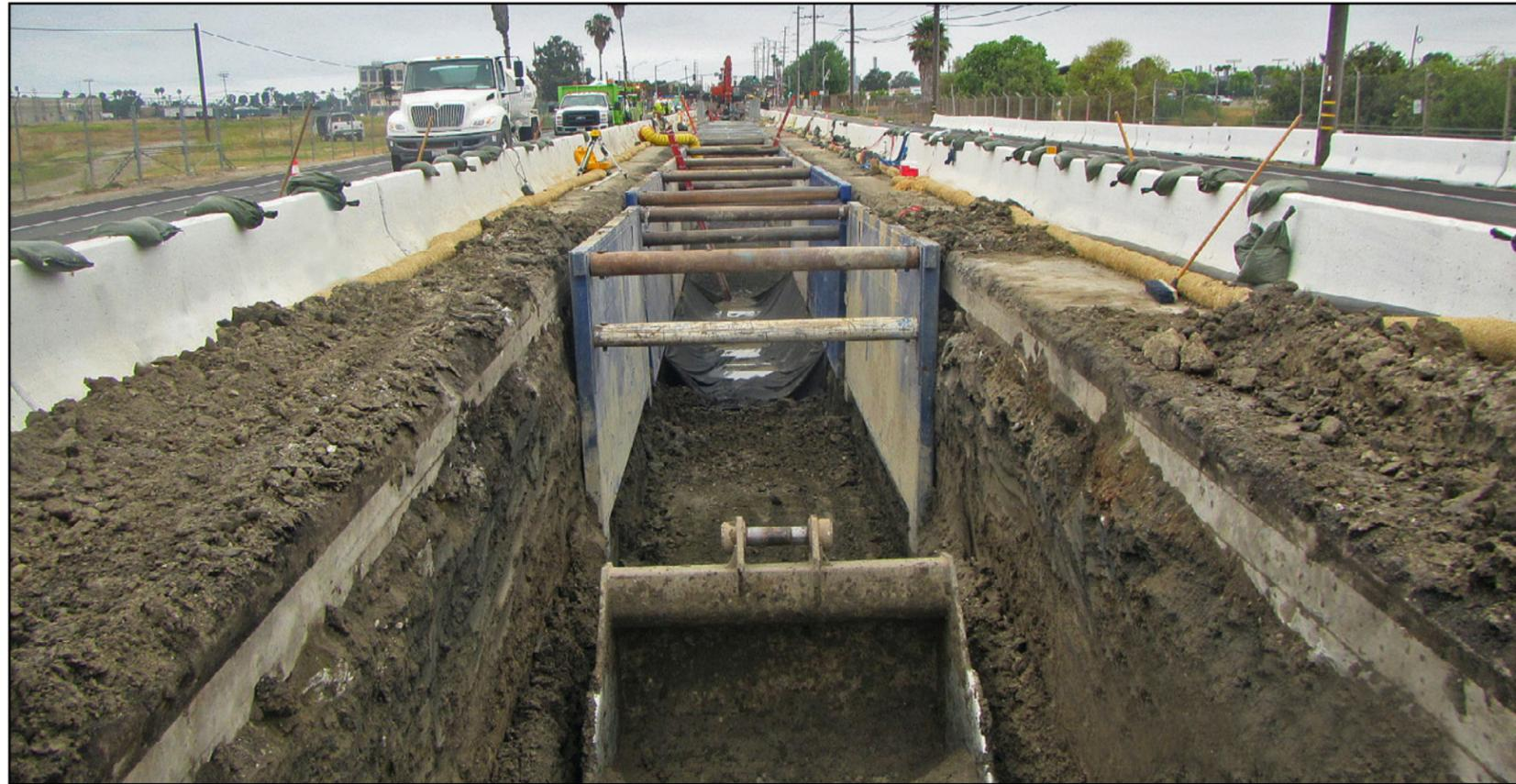
On the Westminster Blvd. Sewer Project, trench shield shoring is used to stabilize the excavation for the dual 36-inch force main pipe installation.
