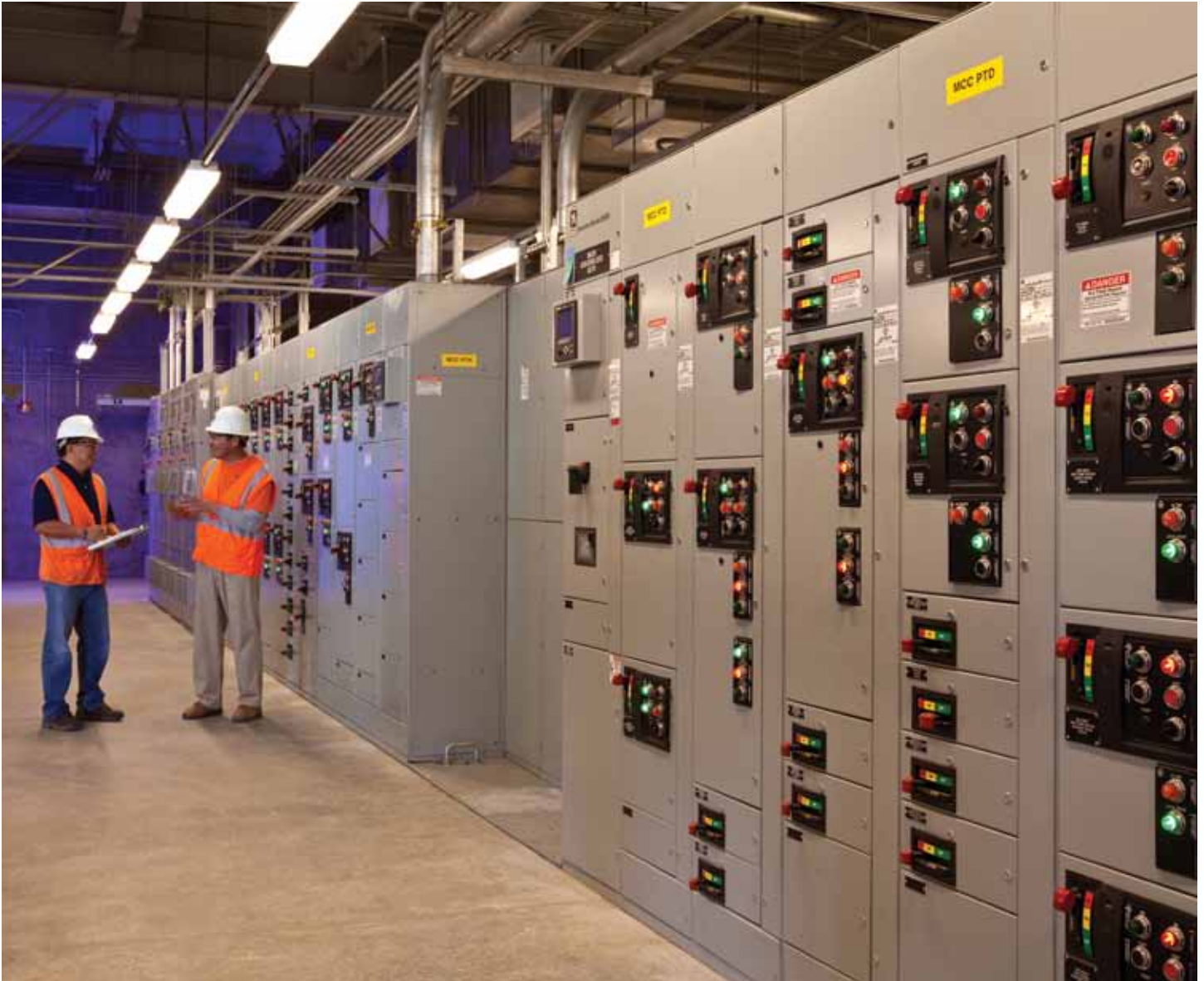
The new Headworks has an extensive power system that incorporates several back-up power options to ensure reliable power delivery to protect the public under unforeseen circumstances.
