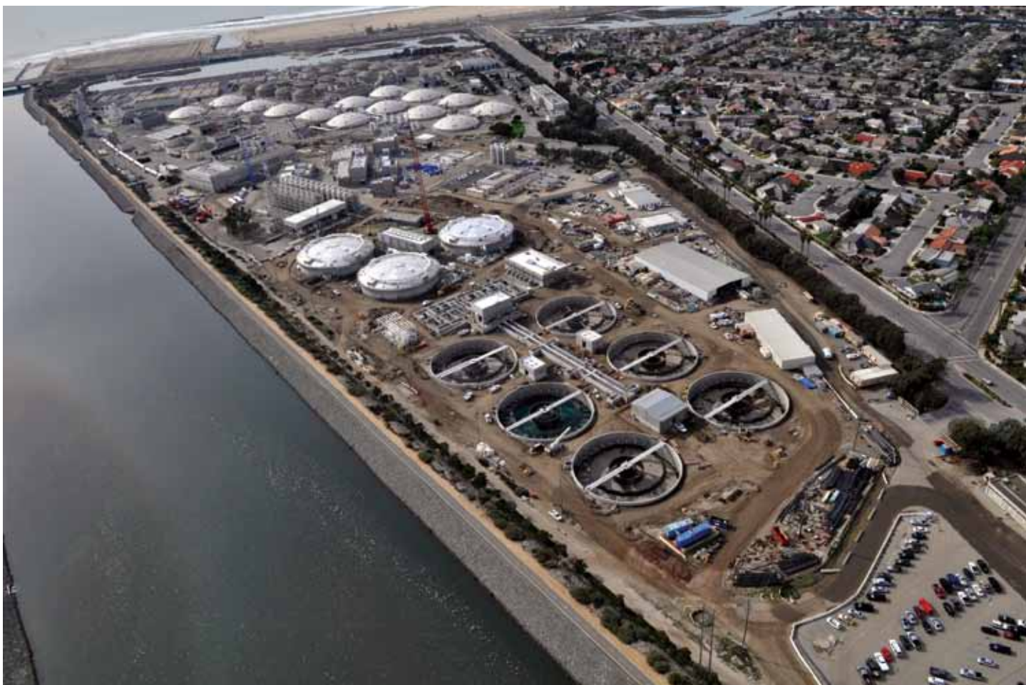
OCCSD's Treatment Plant No. 2 spans 100 acres and borders Brookhurst Street, the Santa Ana River, and Pacific Coast Highway in Huntington Beach, CA.
