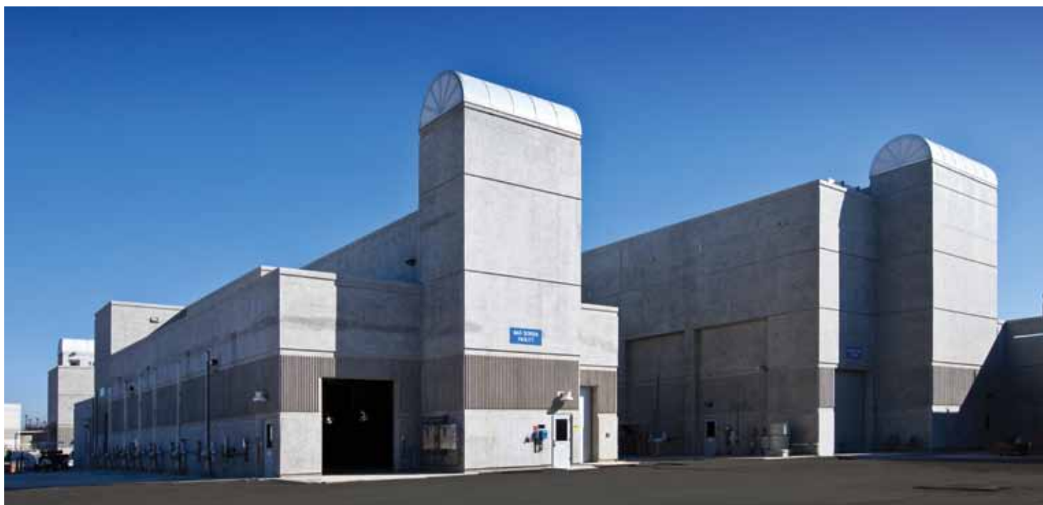
The new Headworks facility at Plant No. 2 pumps all of the wastewater from the collection pipelines into the treatment plant. This facility is currently in testing and being placed into service.
