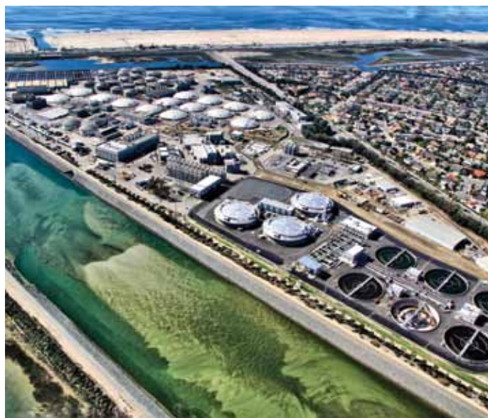
Aerial view of our Huntington Beach Treatment Plant.
