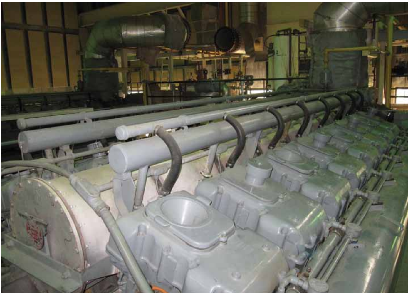
For more than 30 years OCSD has used digester gas (also called biogas, a natural by-product of the treatment process) to fuel our plants to save energy. The Central Power Generation System uses this fuel to power most of the facilities at both plants saving millions in power costs.
